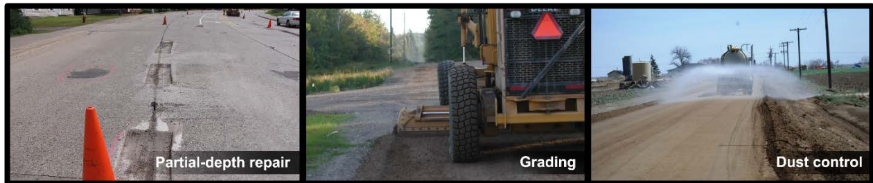
Figure 5: Examples of capital preventive maintenance treatments, cont'd—(from left) concrete road prepared for partial-depth repair, gravel road undergoing maintenance grading, and gravel road receiving dust control application (dust control photo courtesy of Weld County, Colorado, weldgov.com).
