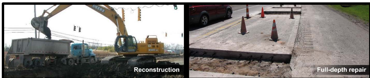
Figure 2: Examples of reconstruction treatments—(left) reconstructing a road and (right) road prepared for full-depth repair.
