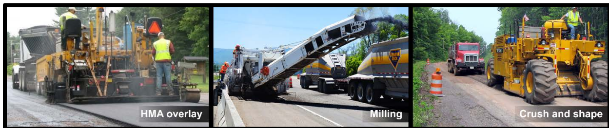
Figure 3: Examples of structural improvement treatments—(from left) HMA overlay on an unmilled pavement, milling asphalt pavement, and pulverization of a road during a crush-and-shape project.
