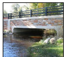
Figure 4: Three-sided box bridge
