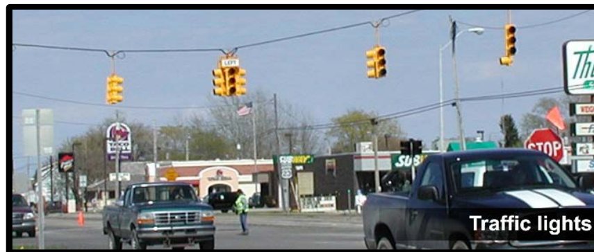
Figure D-1: Example of traffic signals
